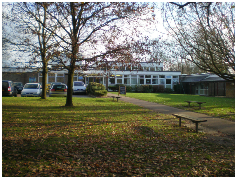
Figure 5 – view showing the existing car park and the two oak trees which would be removed in order to create the car park extension
